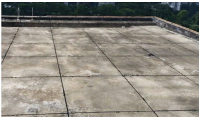
Figure 9: Protected Membrane Roofs in Malaysia
