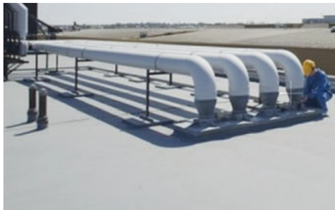
Figure 6: Polymeric coating on the flat roofs
