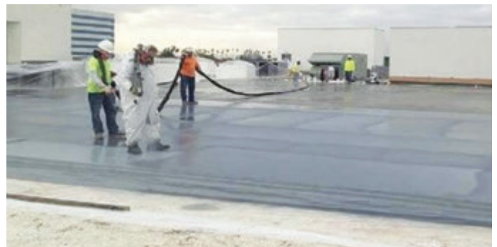
Figure 8: Polyurea waterproofing coating
